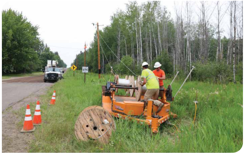
▶ 3 miles of aged line and pole replacements near Saginaw in 2021.
