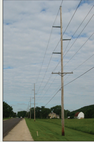
69-kV/115-kV transmission structure with distribution underbuild
