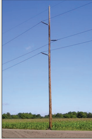
69-kV/115-kV transmission structure
